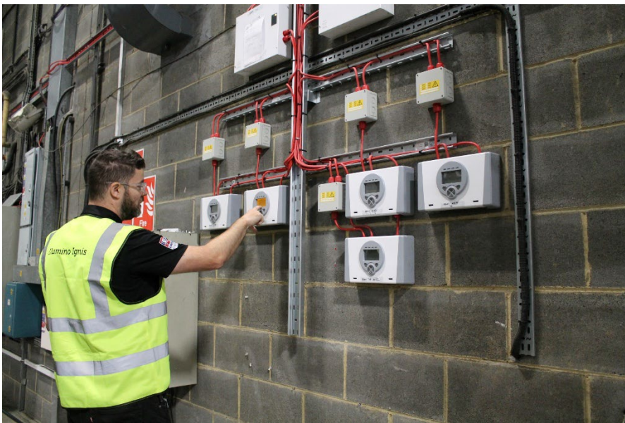
Figure 3: Illumino Ignis engineer commissioning Fireray Hub Reflective controllers at ground level, avoiding repeated
